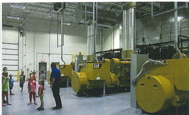
Looking at the generators if we lose electricity, they take over.
