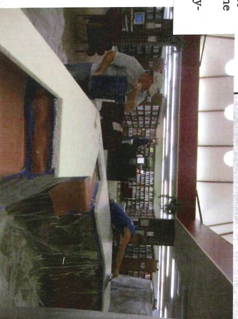
Andy & Rob applying the concrete mixture to the countertops.
