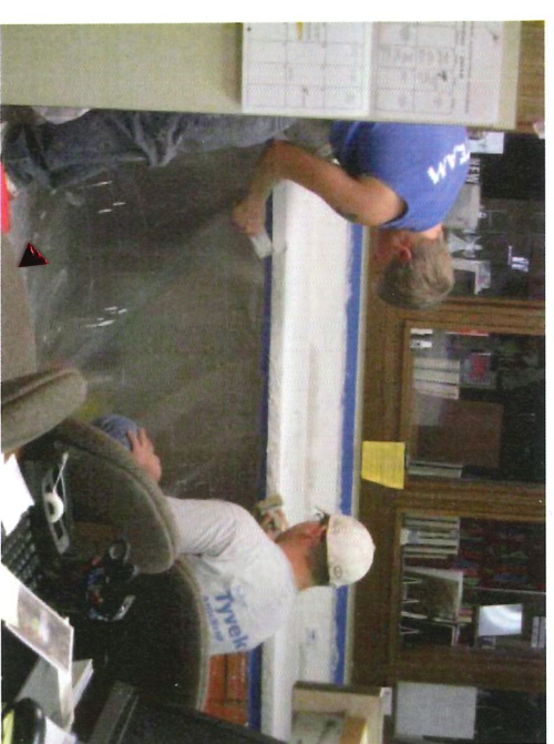
Making the rugged texture on the edges.
