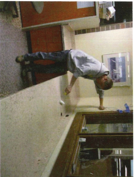
Rob applying the coat of epoxy and two coats of a urethane finish.
