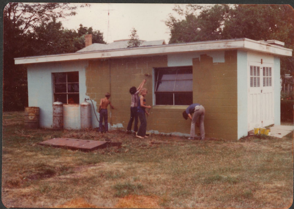
"Before" and "after" pictures of pump house.
